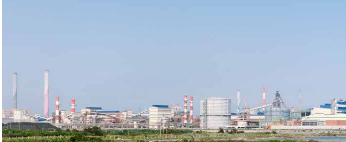
Primetals Technologies takes care of maintenance at the customer's site
