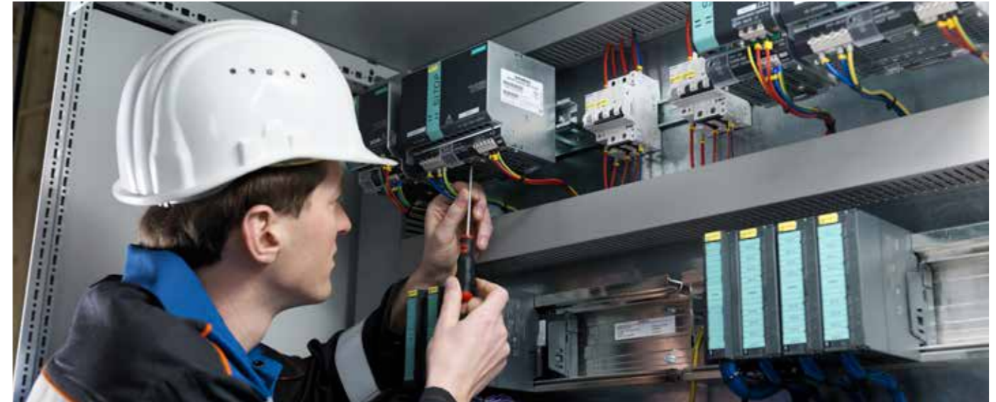
Part replacement in an electrical cabinet
